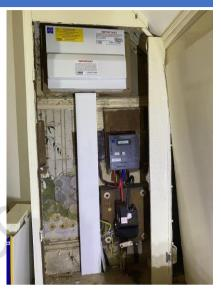
Where before a single RCD was protecting a number of circuits now in order to ensure everything goes off in the right time every circuit needs to have its own separate RCD protection with the use of RCBOs.
