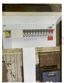
We also had the introduction of Surge Protection Devices (SPDs). What the SPD does is to protect all your electrical devices (Phones, Tablets, Laptops & modern appliances with sensitive electronics in them) in a case of an excess amount of electricity introduced into your electrical installation, most commonly after a lightning strike in the area, But this can also be caused through faulty appliances with any form of motor.
